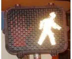
WALK intervals of greater than 7 seconds may be used where the duration of the associated vehicular green interval is long enough to accommodate it. The purpose of the WALK interval is to provide enough time for a group of waiting pedestrians to enter the crosswalk before the flashing DON'T WALK commences.
